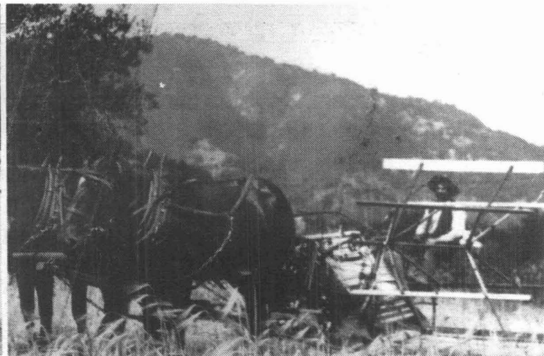
FRED NASON SR., OPERATING his horse-powered wheat binding machine in the Cachagua, about 1920. The binder cut and bound grain into 20-30 lb. bundles, ready for upright shocks.
