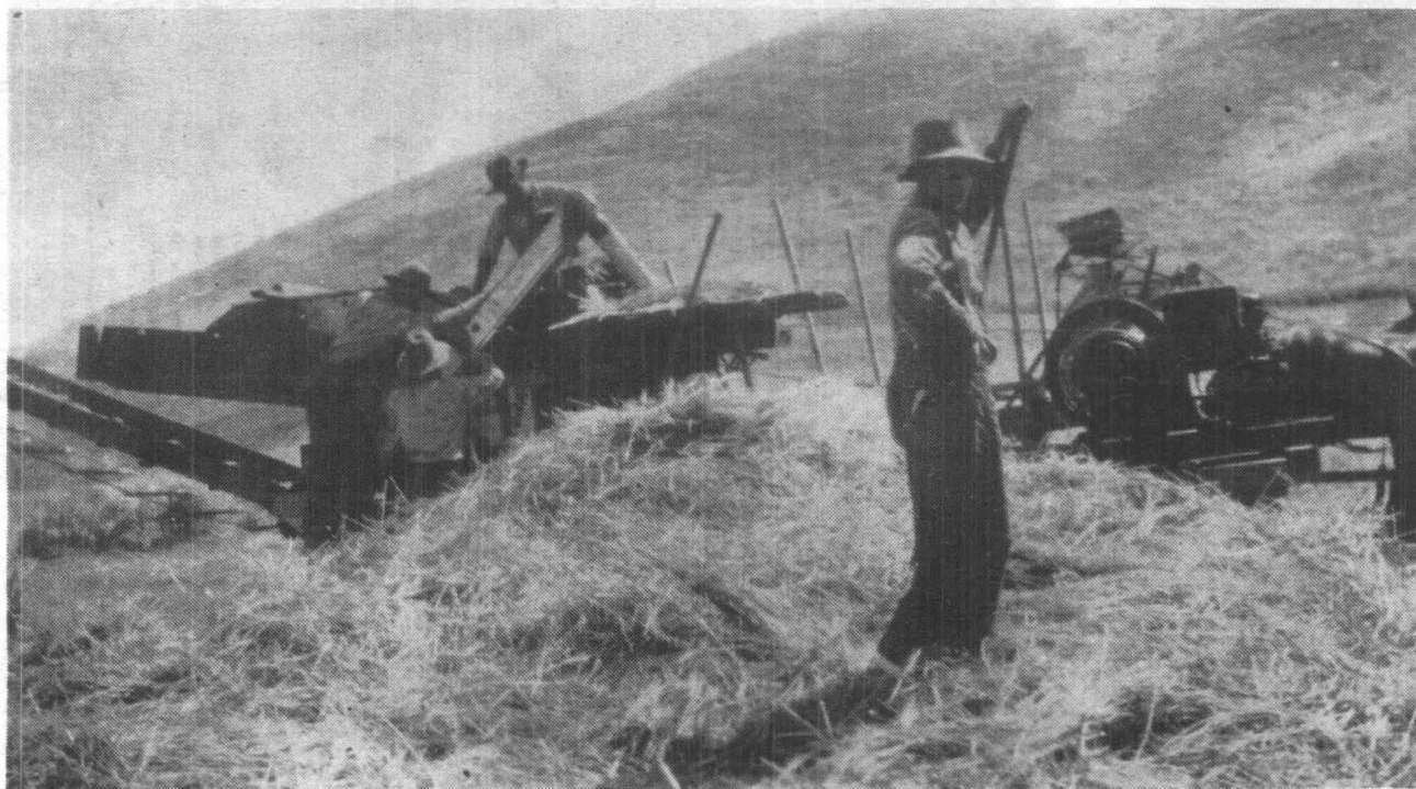
1927 PHOTO of the separator used in those days to thresh barley on the Berta Ranch. Standing in front is John Berta.
